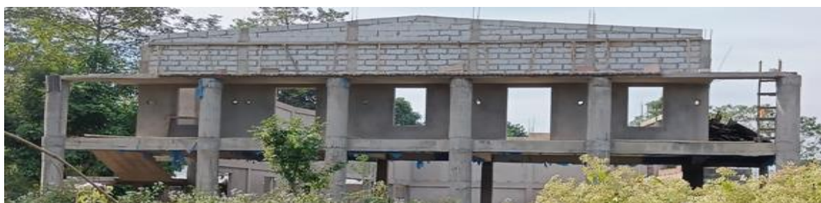
(Construction of University Auditorium is in progress)
